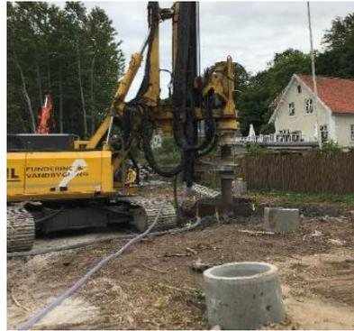
Figure 3. Drill rig 100 ton RTG machine RS20.
