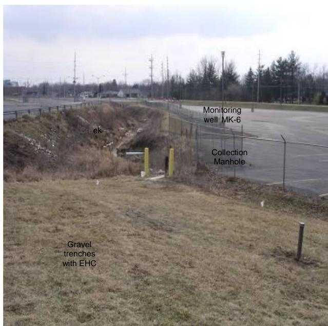
**Figure 8:** Approximate location of gravel trench, manhole CB-1
