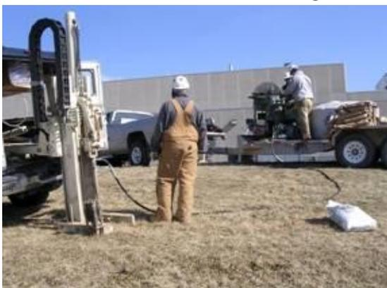
Figure 2: EHC injections at trench along property lines.
